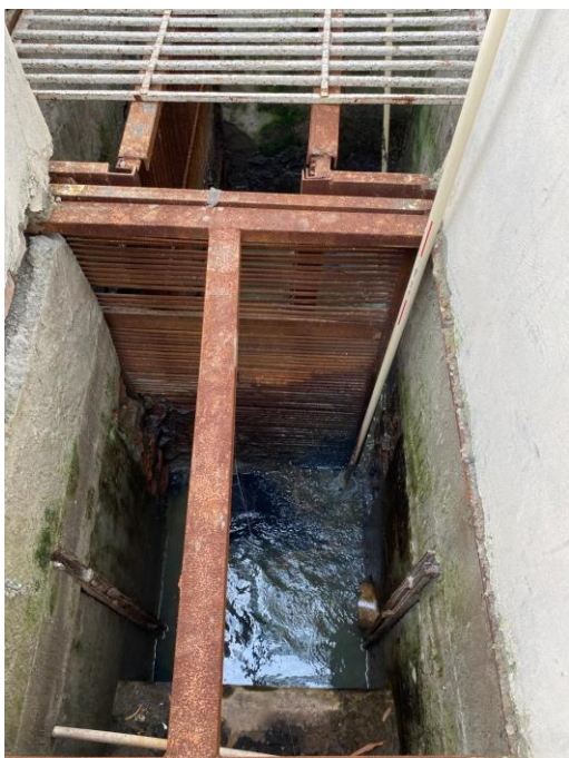
Fig 1.1 This screen filter removes bigger particles from the sewage like paper & plastics
