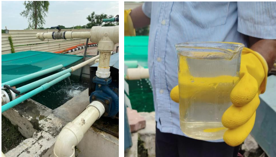
Fig 1.12 exhibits the treated water which is used for irrigation and toilets. It is not fit for drinking
