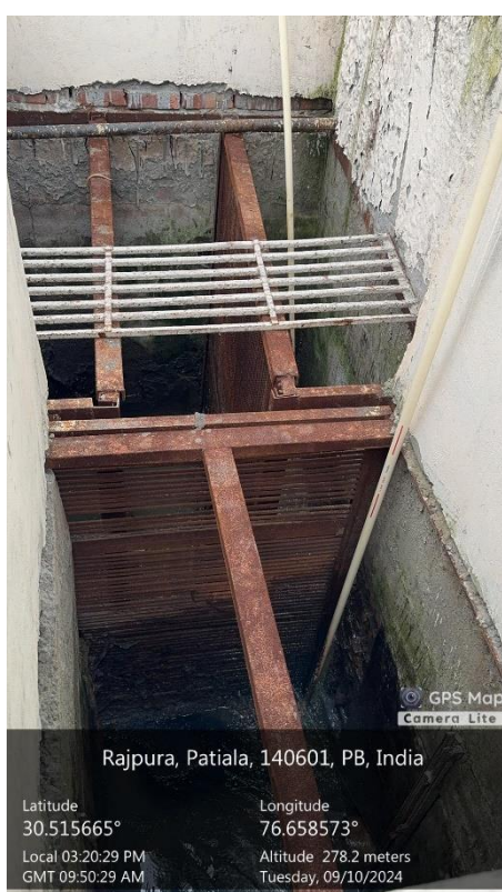
Fig.03: grit for physical separation
